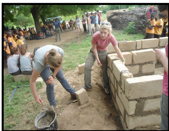
Students laying blocks and plastering the Tampieni primary school urinary
